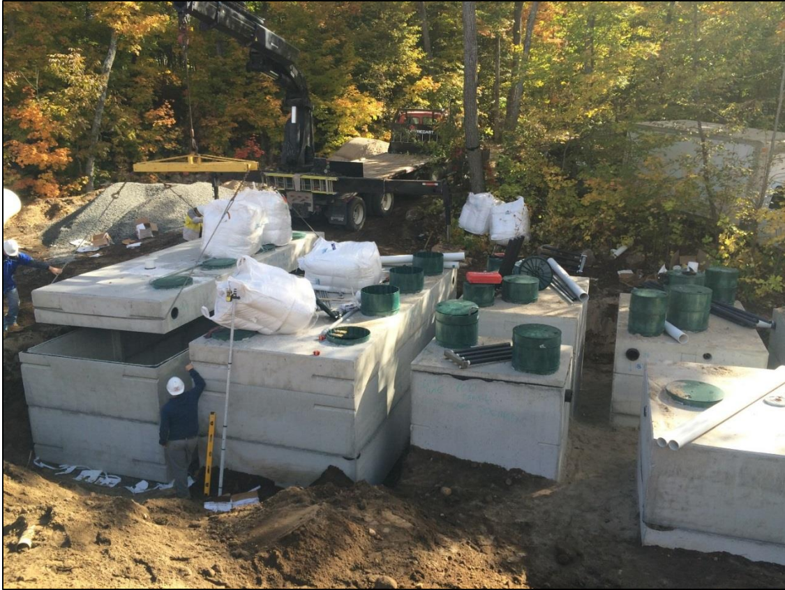
Figure D-1: Installation of a communal wastewater treatment system
