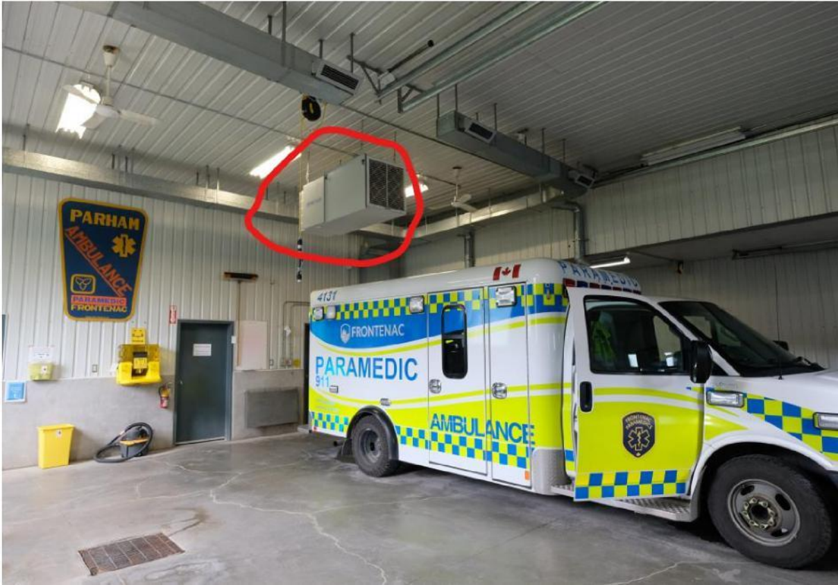
Above: The ceiling-mounted fan unit does not reduce CO.
